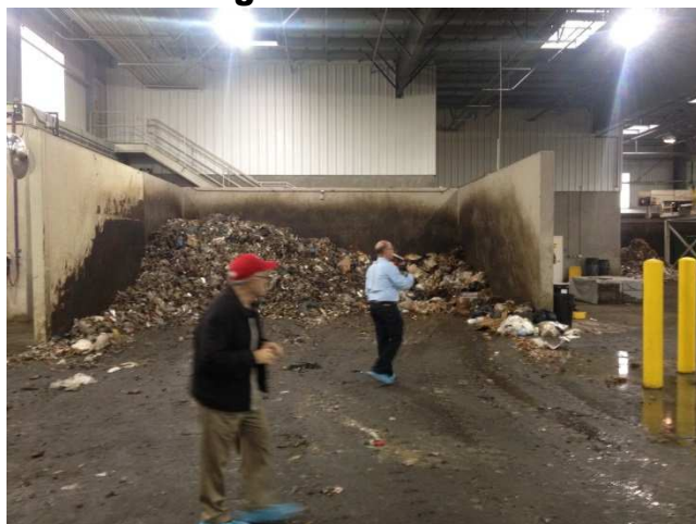
Photograph 1 is a bunker containing organics for the AD system in San Jose. These organics were recovered using MWP equipment.
